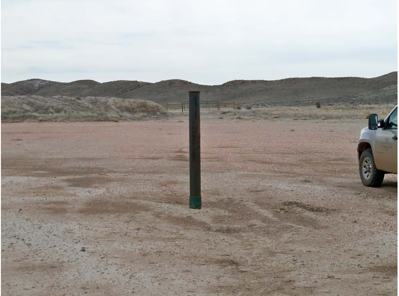
Photograph #4: Evidence of Plugged and Abandoned Well: Pre-Reclamation
