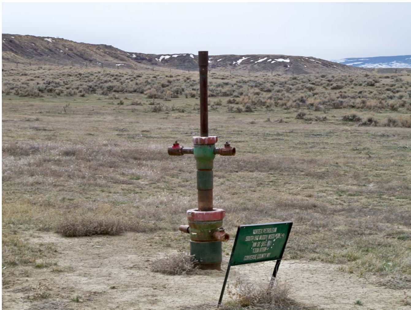
Photograph #1: Non-producing and Bonded Well
