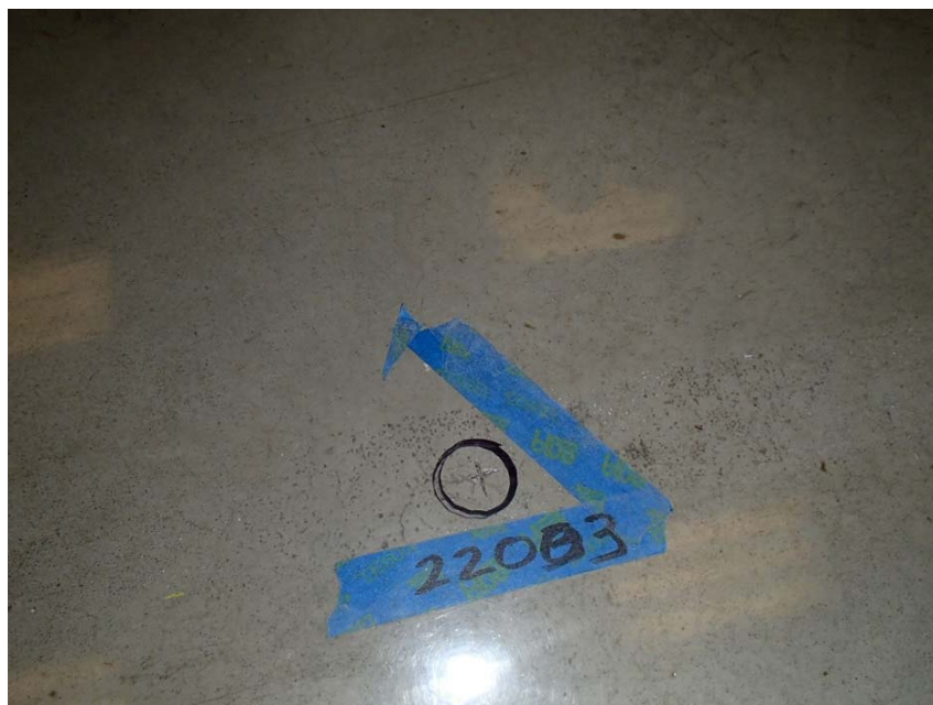
Figure 40. Typical observed control point within the K Unit/Support Building.
