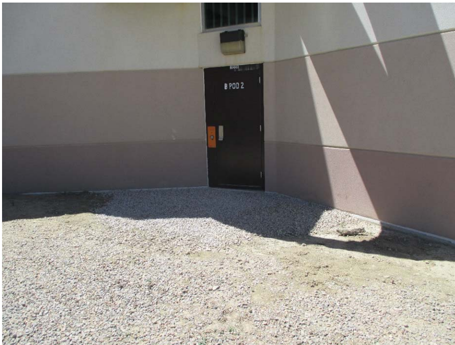
Figure 35. Location where exterior slab was removed and replaced with gravel.
