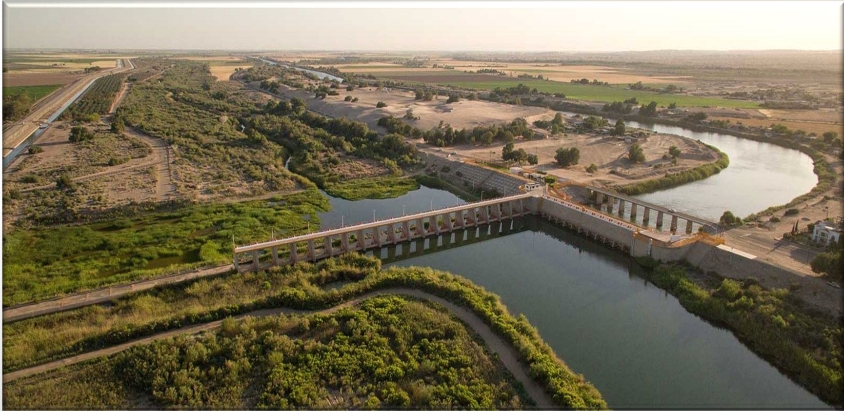
Morelos Dam, Northern International Boundary
