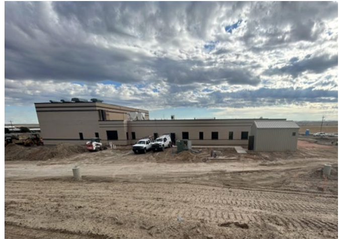
Campbell County School District #1 Little Powder K-8 Back, gym wing.
