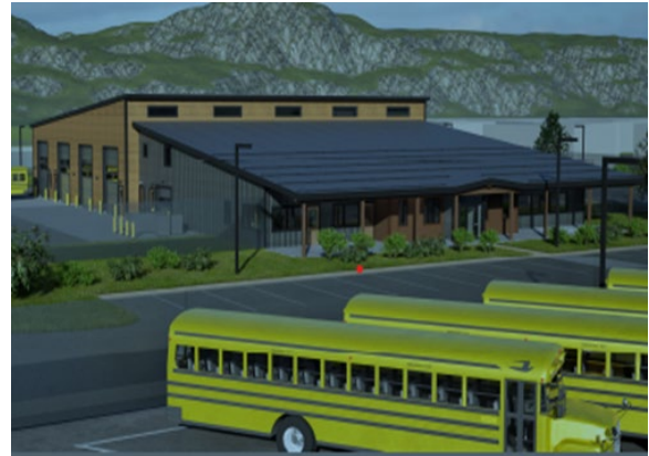
Teton County School District #1 Transportation Facility
