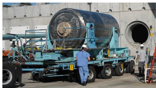
Workers prepare to load an AREVA-TN NUHOMS canister into a concrete storage module at the Calvert Cliffs Nuclear Power Plant in Lusby, MD. (Courtesy: Exelon)
