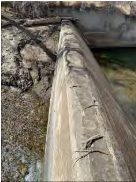
Spillway Diversion on Sybille Ck Backs up water for Canal 1 Headgate
