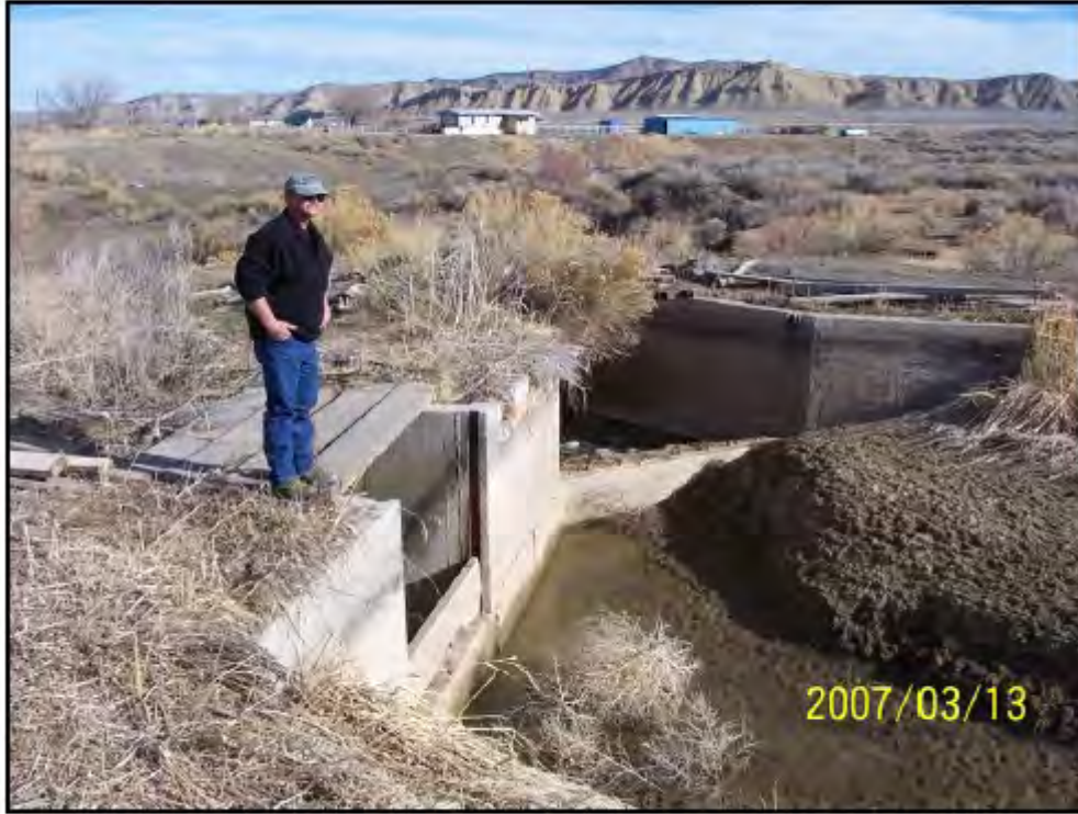
Figure 1.3 Kirby Creek Siphon Inlet.
