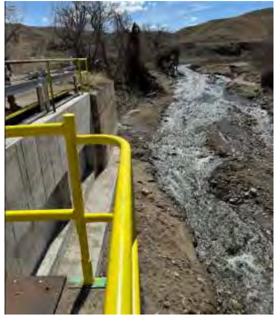
Canal 1 Headgate off Sybille Ck
