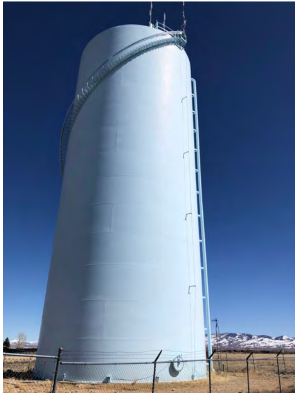
Existing Welded Steel Tank
