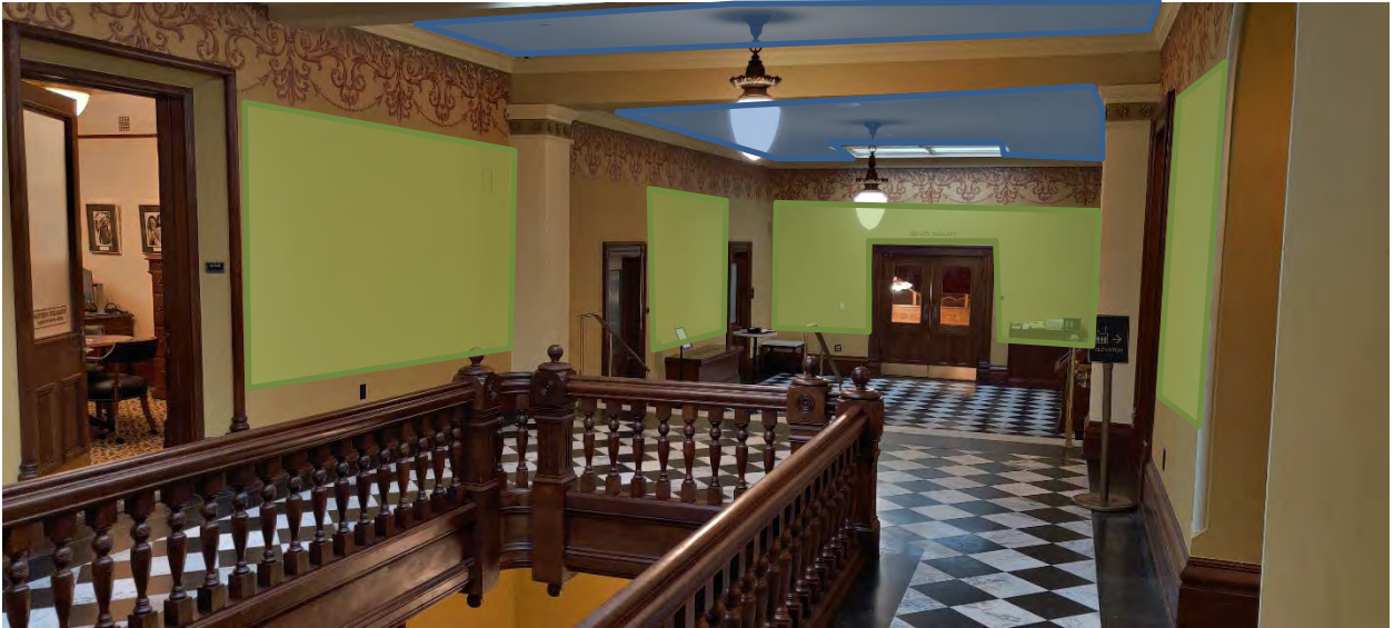
Figure 26. Recommended sound absorption installation locations. Typical for Level 3. Recommendation is for ceiling absorption or wall absorption.
