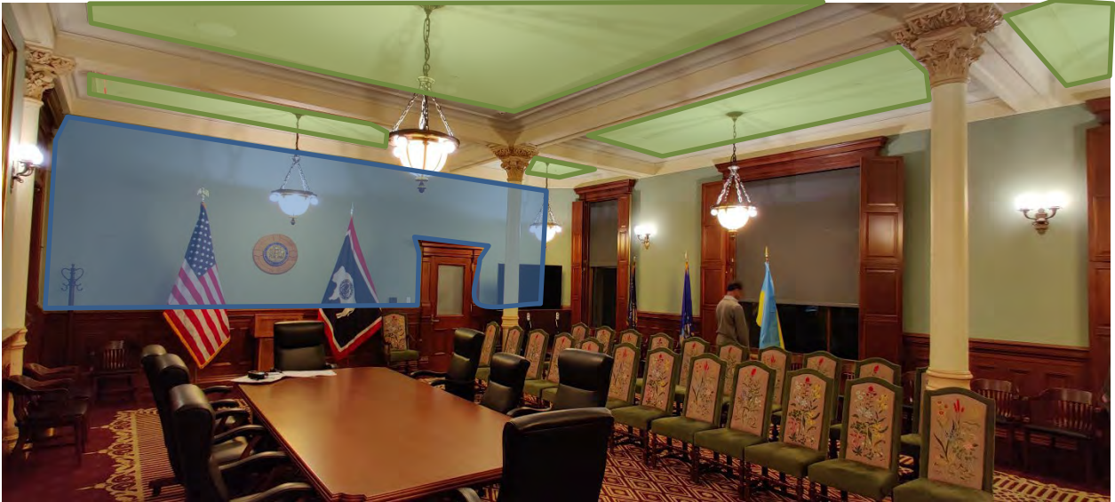
Figure 22. Recommended locations for wall or ceiling mounted sound absorption. Layout would be similar on other walls or ceiling areas not shown.
