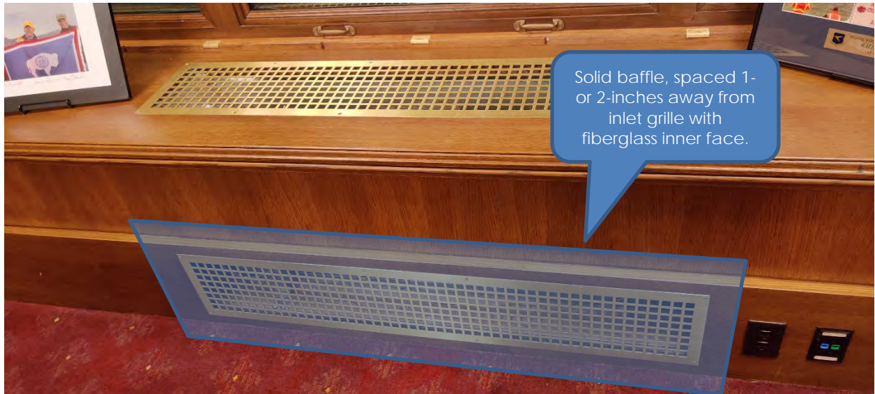
Figure 33. Fan Coil Unit inlet baffle diagram.
