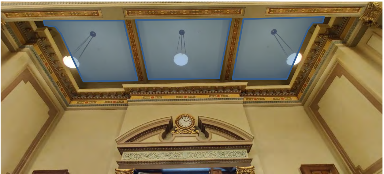
Figure 6. Recommended location for additional ceiling mounted sound absorption.
