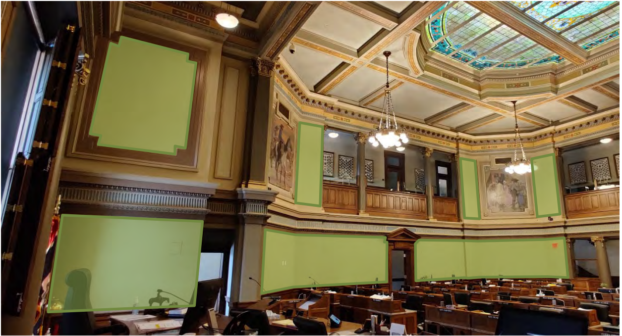
Figure 5. Recommended locations for wall mounted sound absorption. Layout would be similar on other walls not shown.
