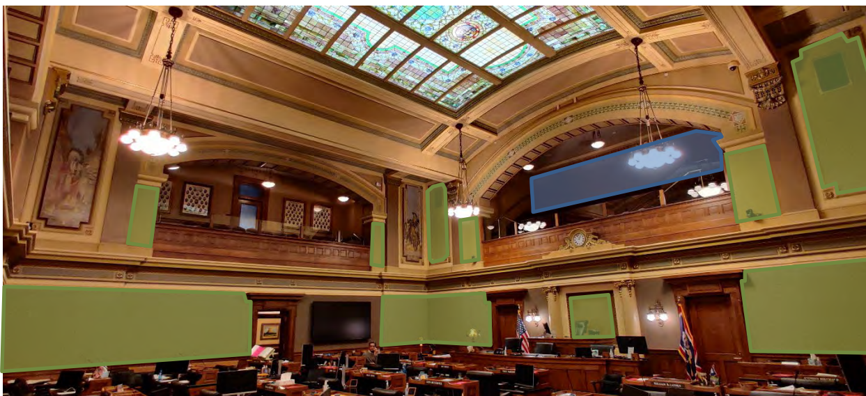
Figure 9. Recommended locations for wall mounted sound absorption. Layout would be similar on other walls not shown.
