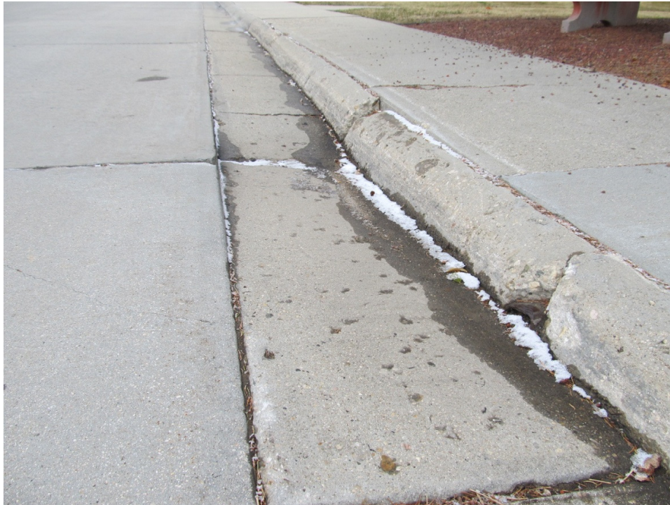
Figure 2.1.5: VHW Settled curb and gutter section
