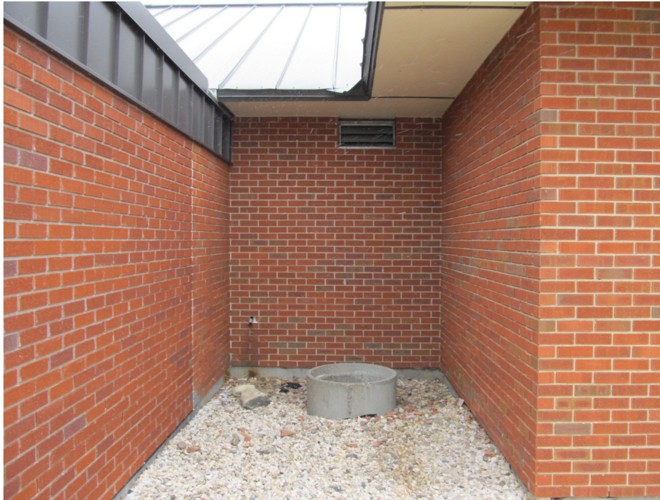
Figure 2.1.3: VHW Vertical concrete pipe section used to catch roof run-off
