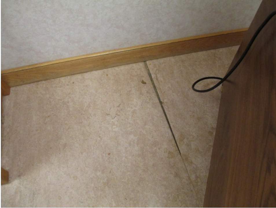
Figure 3.4.8 VHW Linoleum flooring with split seam
