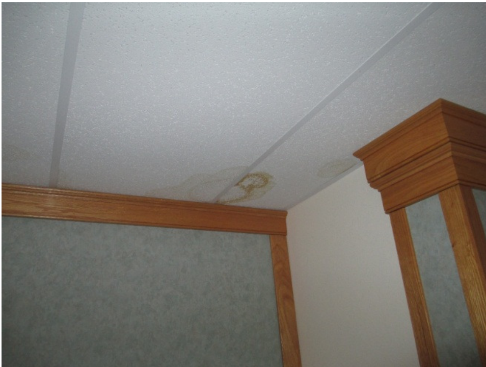
Figure 3.4.9: VHW Roof Leak
