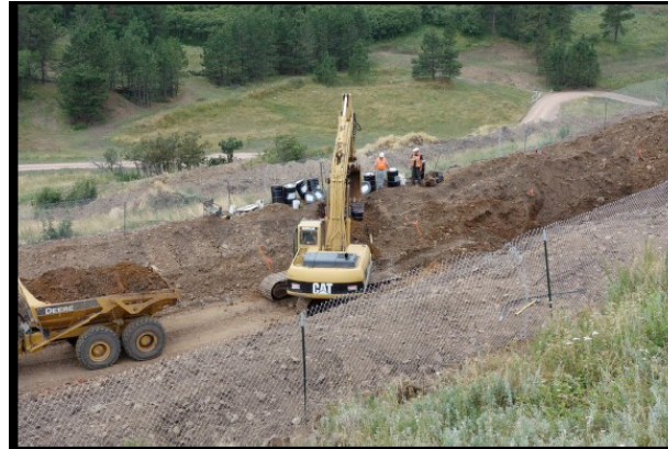
Trench exposed near-surface main dyke and was bulk sampled along 300 foot length Trench reclaimed in 2015
