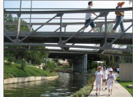
Pedestrian overpasses and underpasses allow for the uninterrupted flow of pedestrian movement separate from vehicle traffic. Source: pedbikeimages.org - Julia Diana (2009)
