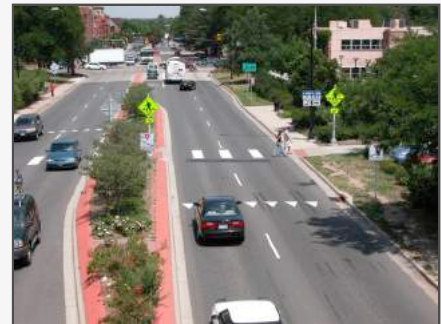
Advance yield markings at a midblock crosswalk with a refuge island. pedbikeimages.org - Toole Design Group.
