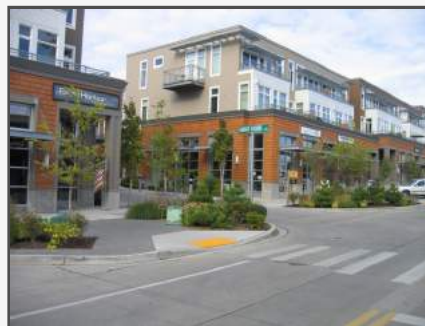
This curb extension at an intersection shortens the crossing distance for pedestrians and creates space for landscaping. pedbikeimages.org - Carl Sundstrom
