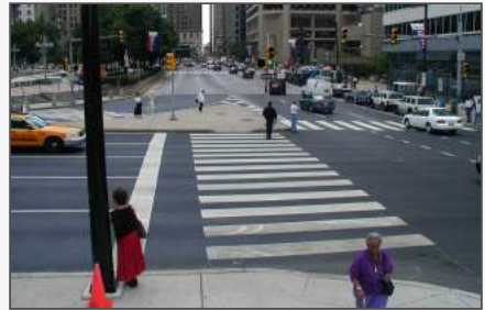
Crossing islands can be located at intersections or midblock crossings to help protect crossing pedestrians from motor vehicles. They and allows pedestrians to avoid conflicts with traffic at street level. Source: Designing for Pedestrian Safety
