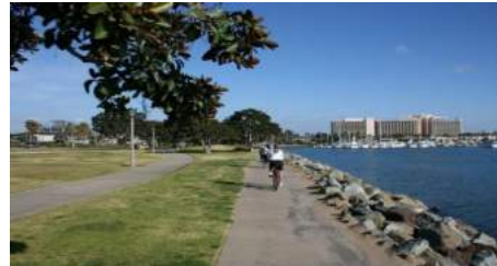
Figure 3: Bikeway (Concrete Bicycle Path)
