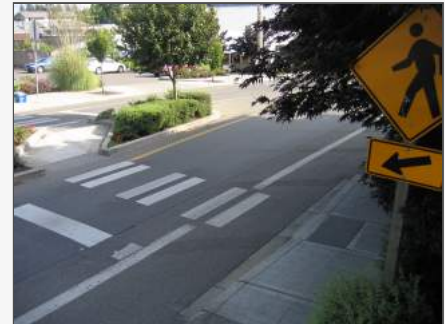
A marked crosswalk with a warning sign and pedestrian refuge island. pedbikeimages.org - Carl Sundstrom
