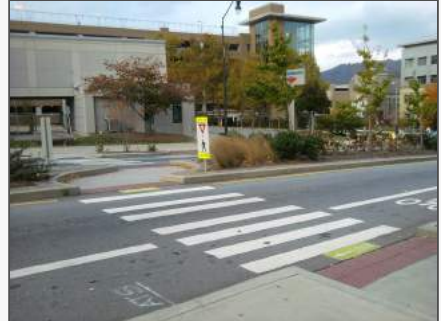
Center crossing islands allow pedestrians to deal with only one direction of traffic at a time, and can be constructed so that crossing pedestrians are forced to the right to view oncoming traffic as they are halfway through the crossing. Source: pedbikeimages.org - Lyubov Zuyeva (2011)
