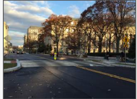
This midblock raised pedestrian crossing features curb extensions and an in-street pedestrian crossing sign. Pennsylvania Department of Transportation.
