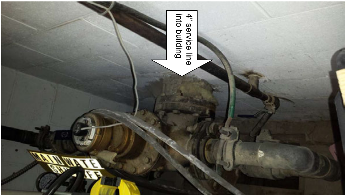
Combined water/fire service through basement mechanical room wall
