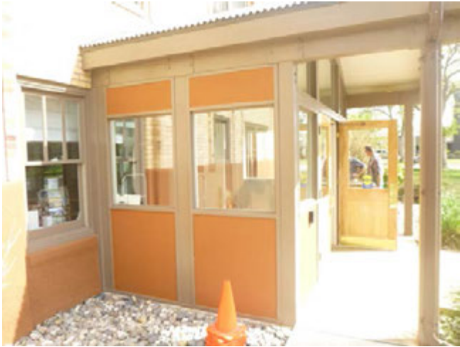
View of entry post and beam structure with infill wall and windows visible (Item S13).
