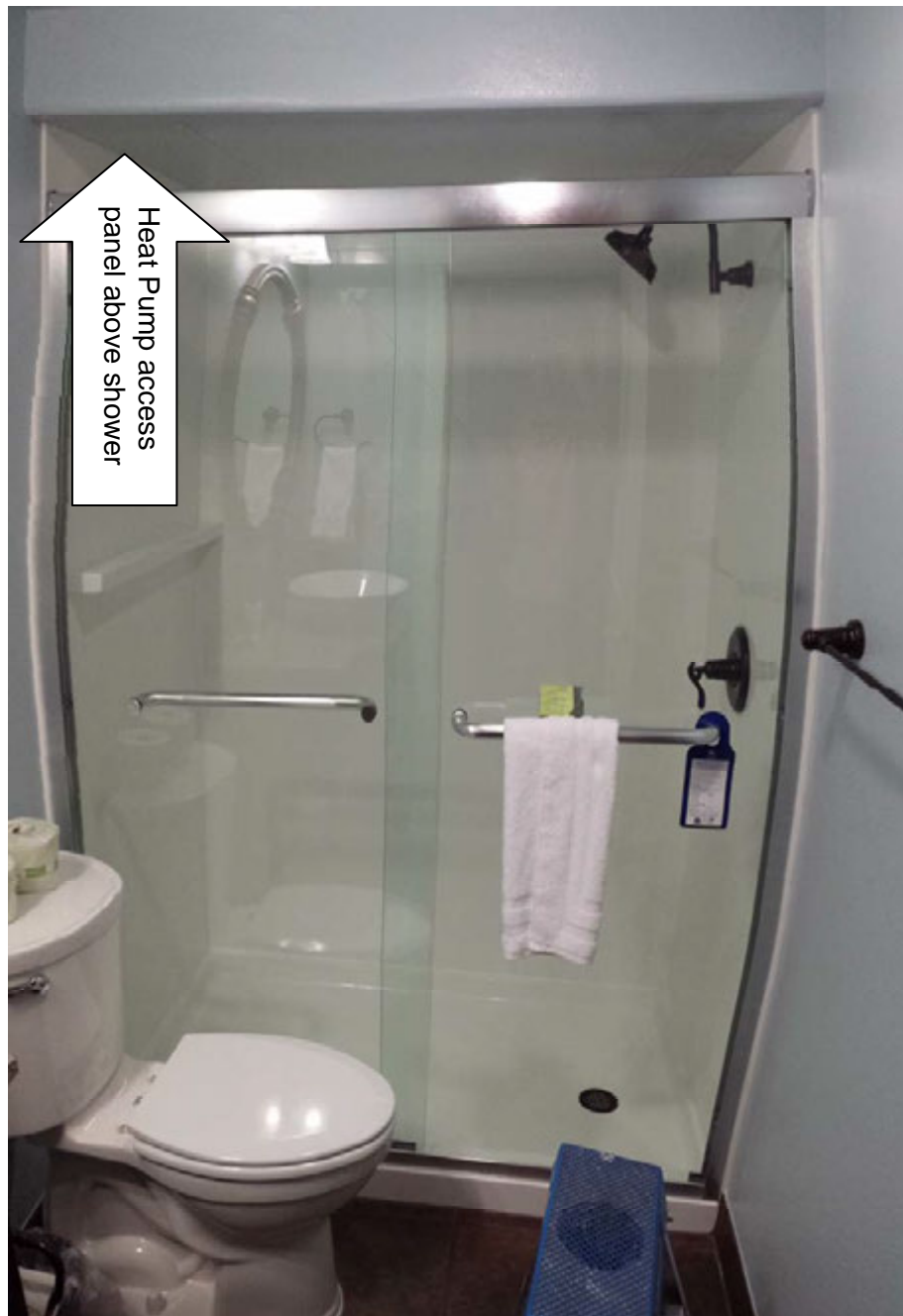
Heat pump inaccessible without removing shower door and frame.
