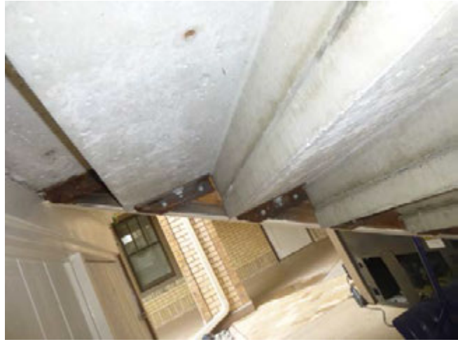
View exterior concrete stair treads and connection to glulam wood stringers (Item S12).
