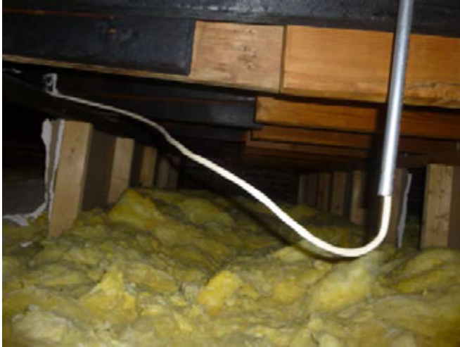
View of roof framing with charred wood visible from past fire (Item S8).
