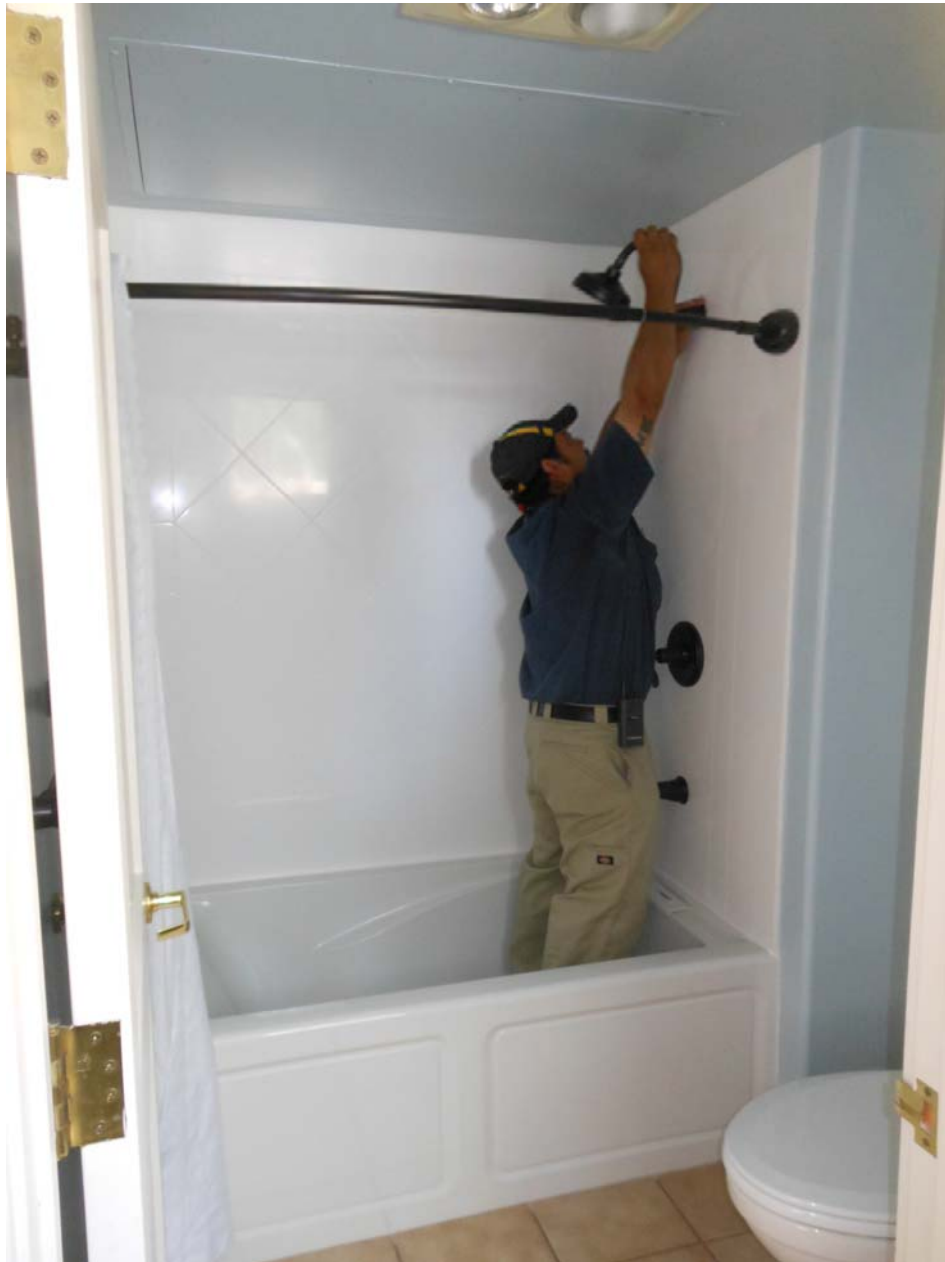
Heat pump access in rooms with tubs requires removal of shower head and arm.
