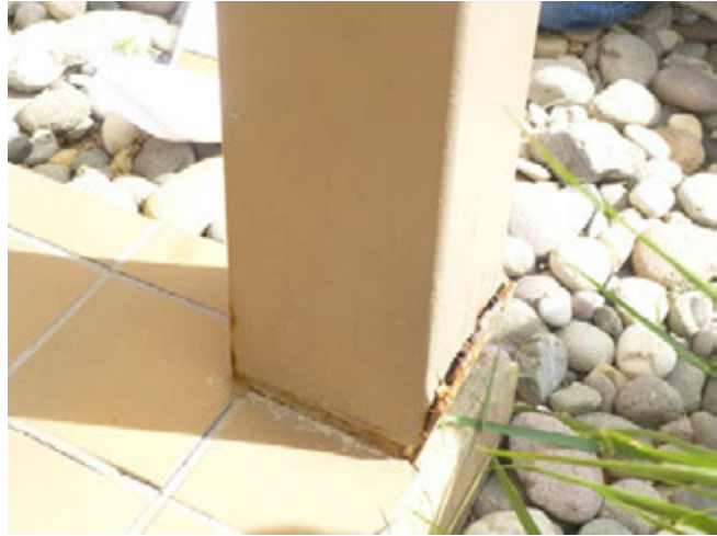
View of corrosion at entry post base connection (Item S13).
