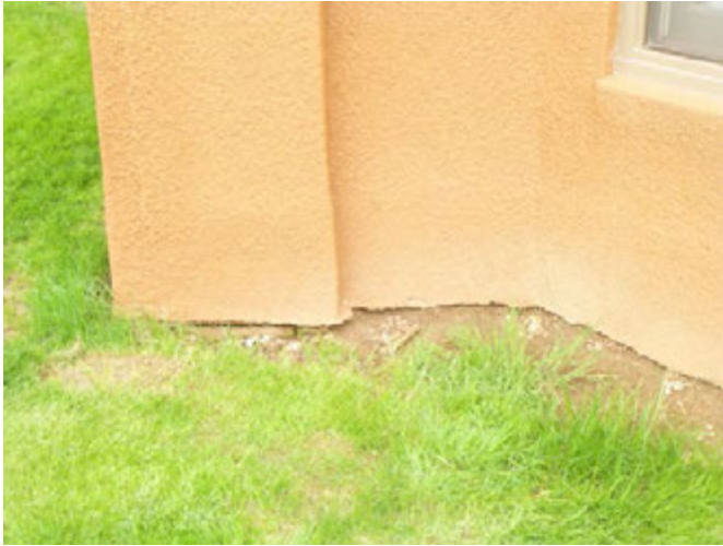
View of typical site grading around building with potentially poor drainage (Item S4).
