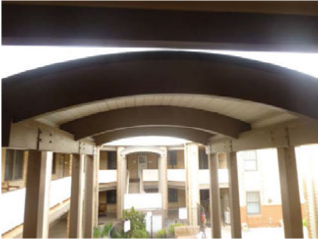
View of roof framing over stairs and wood post supports (Item S10).
