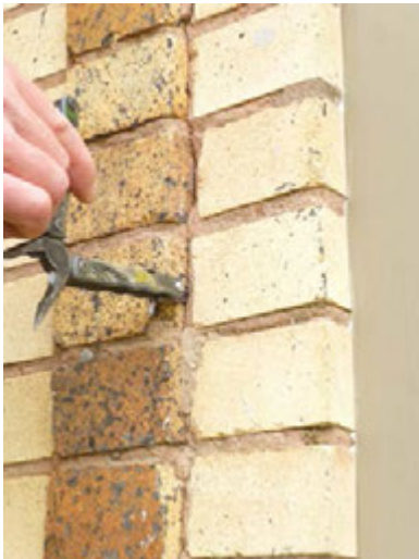
View of soft mortar joints at exterior walls (Item S10).
