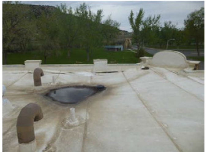
View roof membrane with standing water visible (Item S8).
