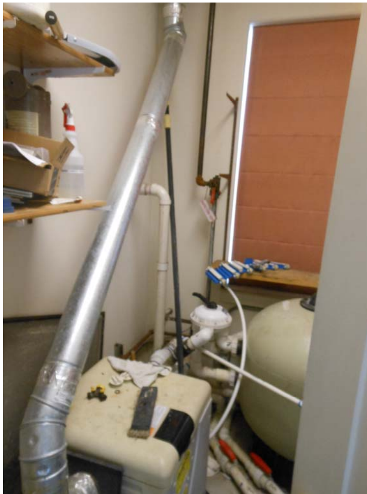
Pool heater and venting
