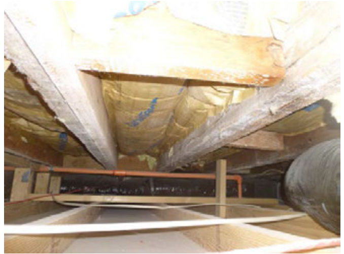
View upper floor framing exposed above dropped ceilings (Item S6).
