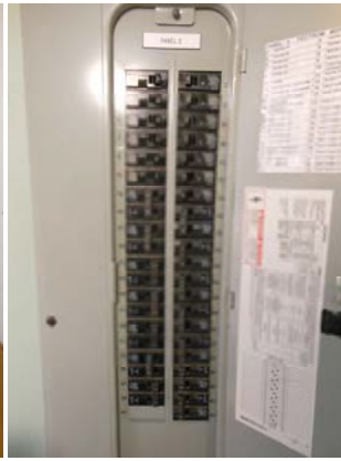
Typical Load Center Panel
