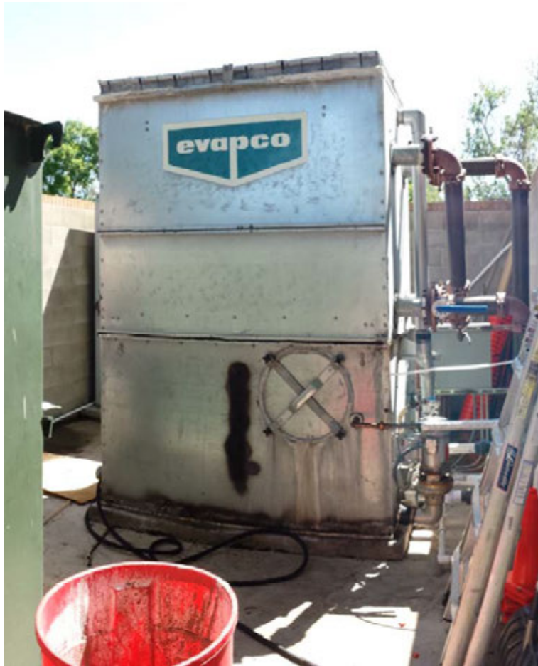
Fluid Cooler for Heat Pump System
