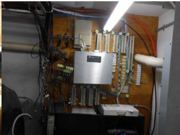
TBB, phone switch and TV splitters
