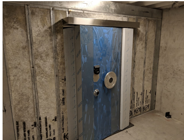
BitGo's Class III bank-grade vault (under construction)
