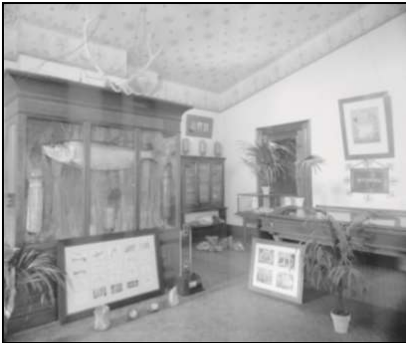
Historic Photograph of Room 302 with Decorative Paint on Vaulted Ceiling
