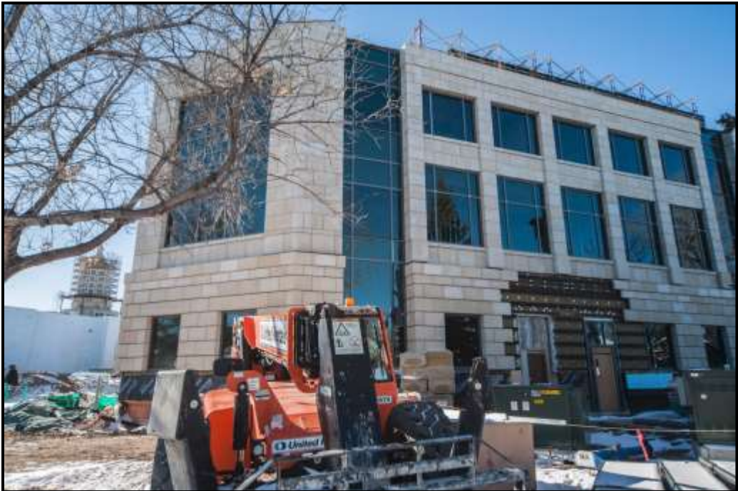
New Steel Framing for Expansion of Herschler Building to the South
