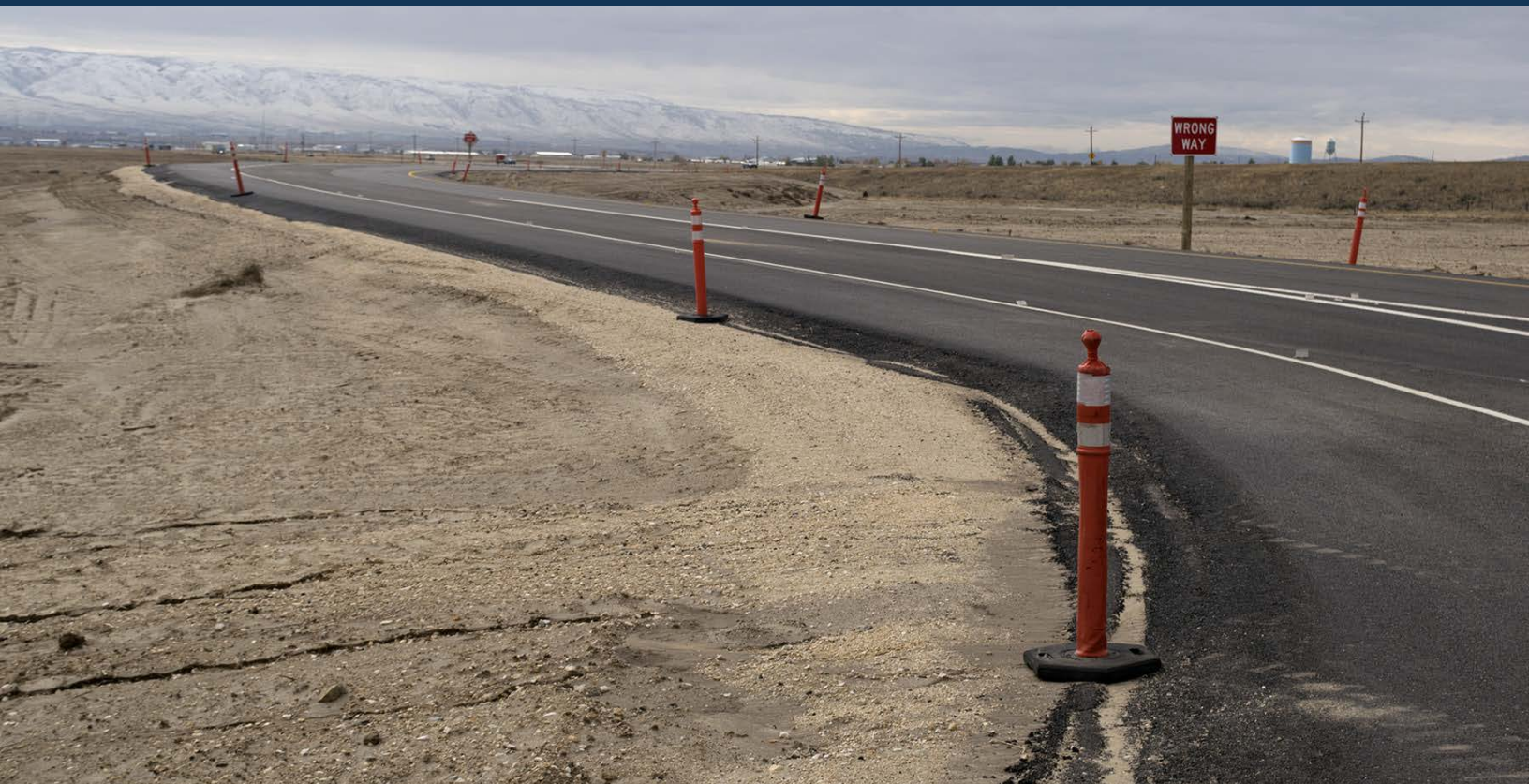
Above: Northbound off ramp.
