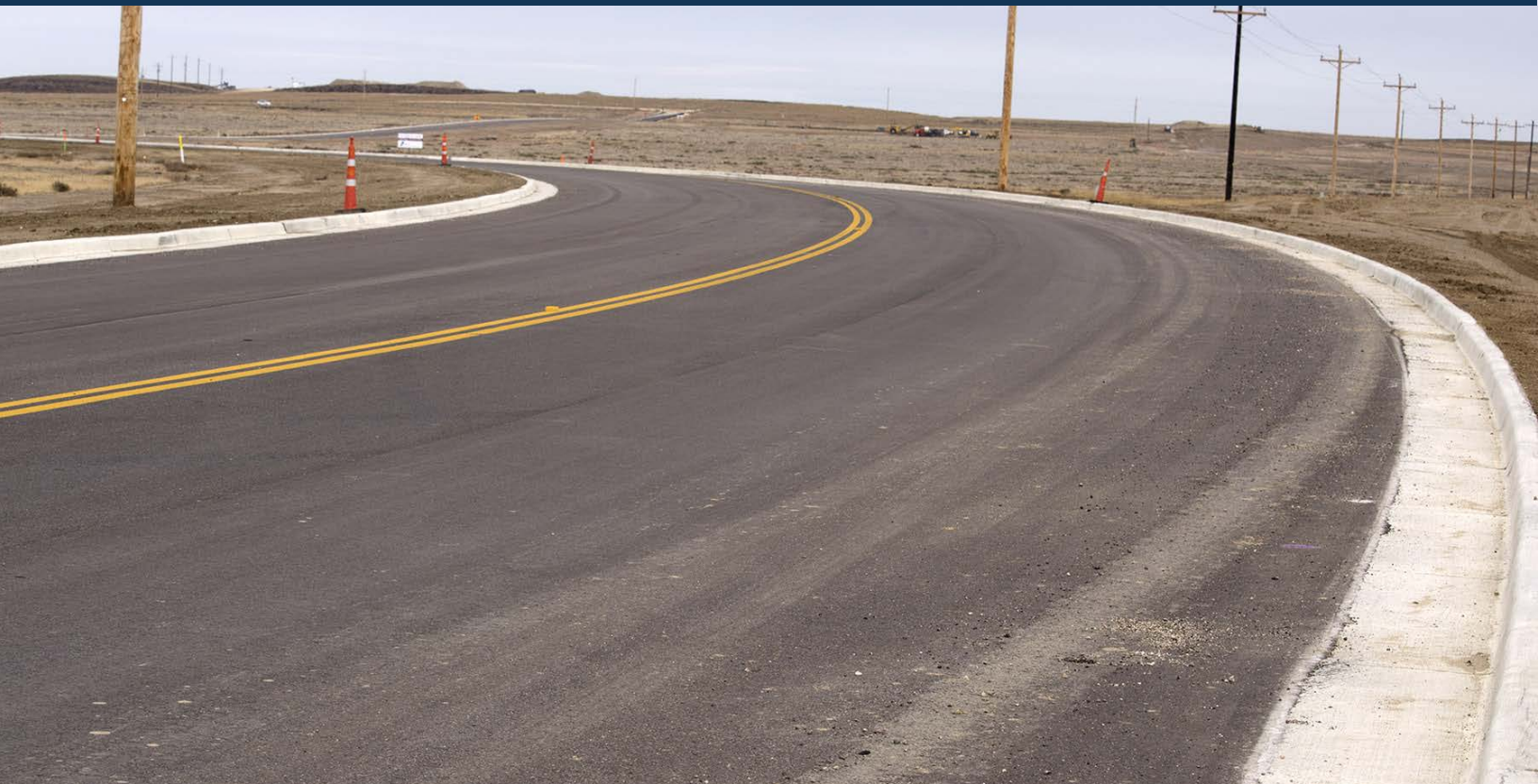
Above: Salt Creek Highway northbound.
