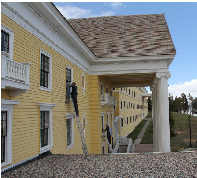
Rehabilitation project (2014). Dick Anderson carpenters installing newly restored window sash and new historically accurate window screens. Photograph courtesy of Yellowstone National Park.
