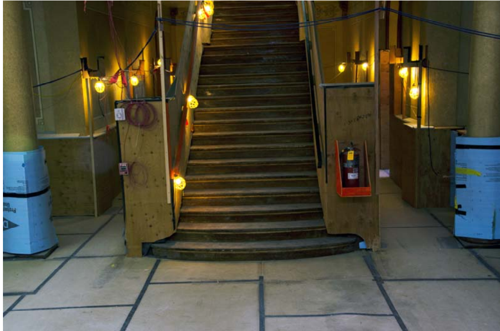
First Floor Grand Stairs
