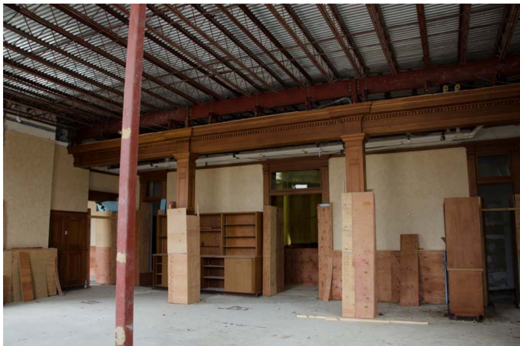
Second Floor Demolition (Supreme Court Space)
