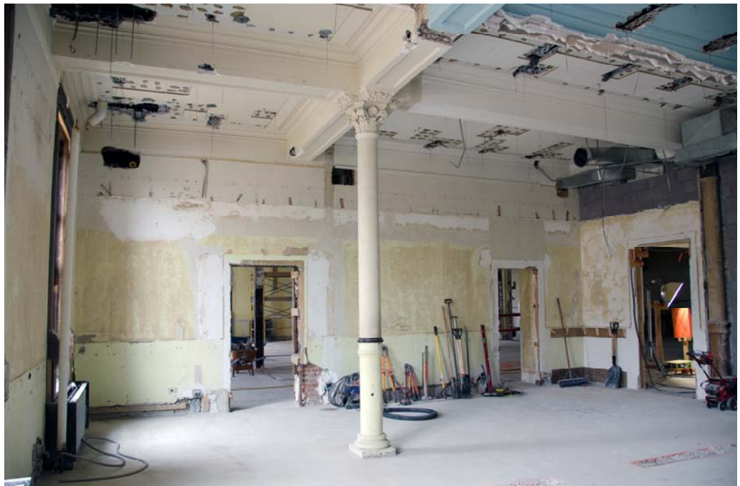
First Level Demolition
