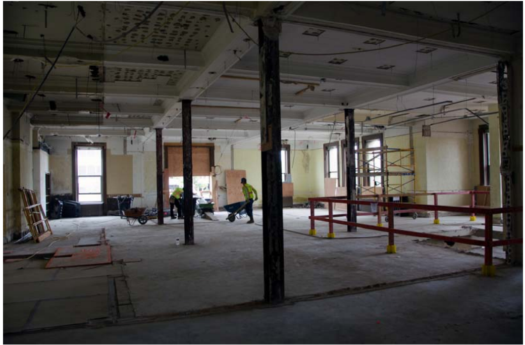
First Level Demolition
