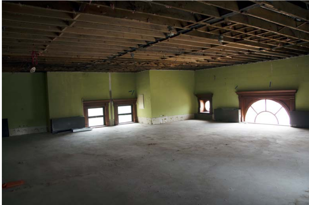
Third Floor Demolition of the Supreme Court Space
