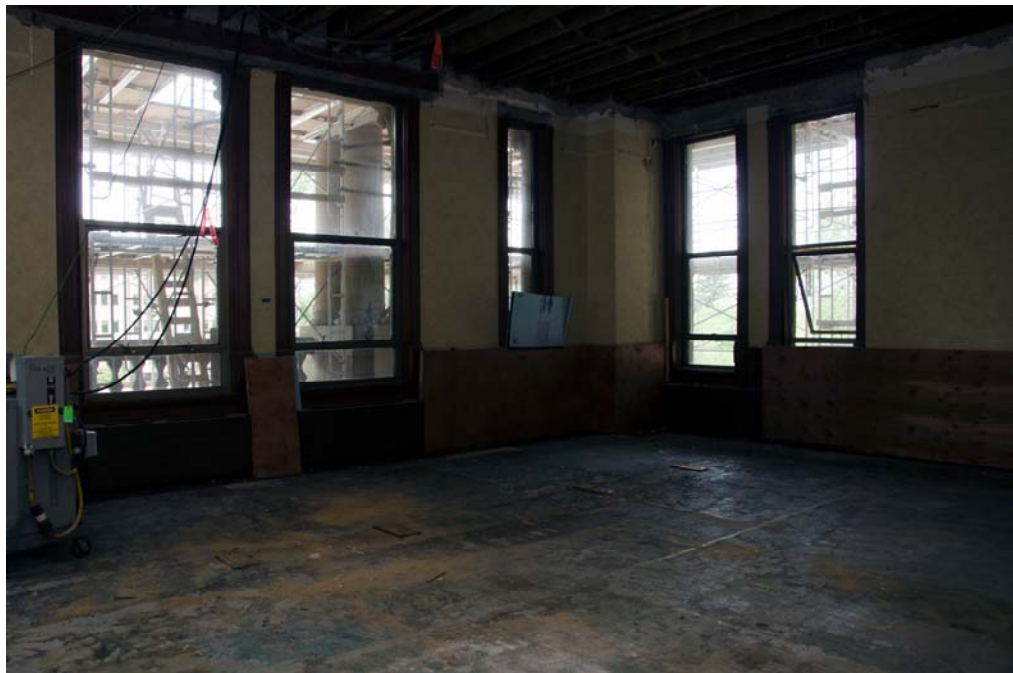
Second Floor Demolition
