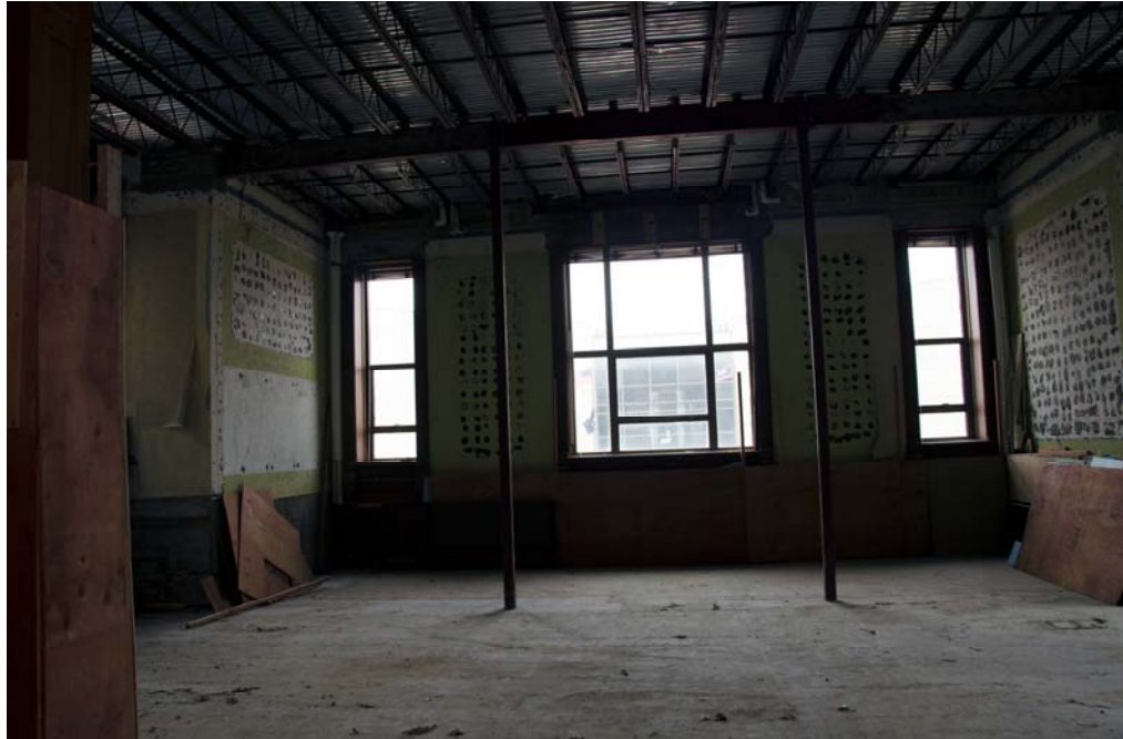
Second Floor Demolition (Supreme Court Space)
