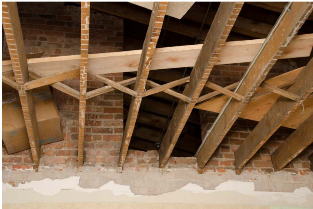
Third Floor Ceiling Demolition
